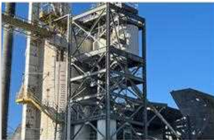
Equipment Fabrication & Erection
