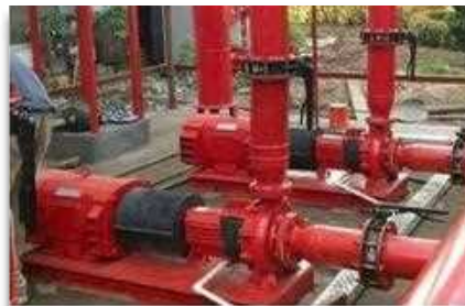
Firehydrant Line Work
