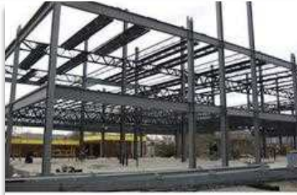
Convention Building / Fabrication Erection
