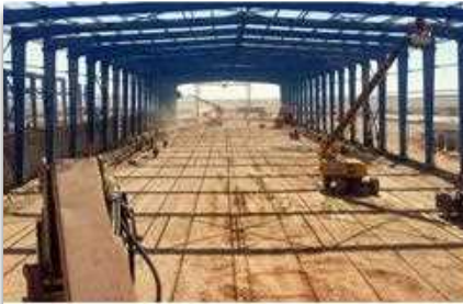
Pre Engineered Building Fabrication Erection
