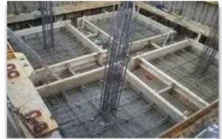
Civil Foundation Work
